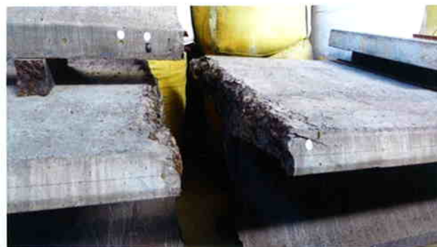
Figure 1: High strength ductile concrete loaded to failure
