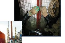
Cutaway view showing the original concrete pile and the new SPT FABRICFORM Pile Jacket
