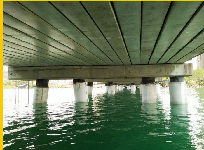
Pile Protection Works for Wharves
