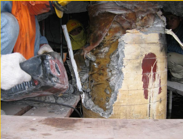
Pile Restoration Works for Passenger Jetty
