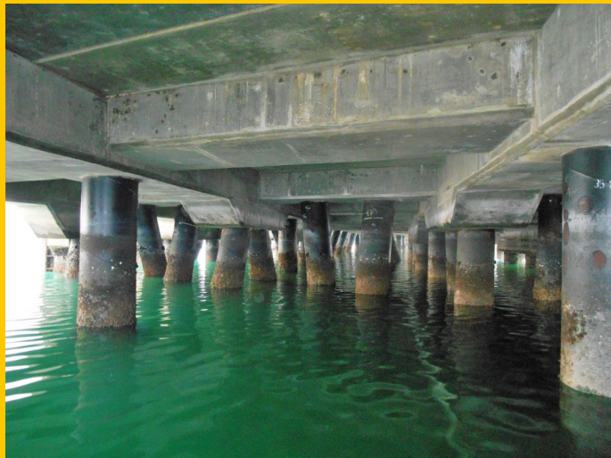
Pile Protection Works for Wharves
